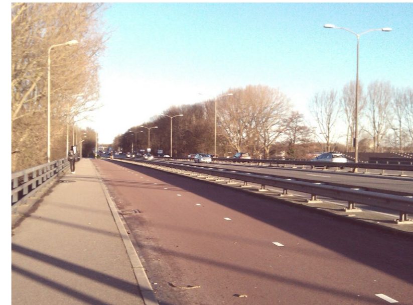
Figure 80. Total separation of flows. Pedestrian sidewalk, cyclist lane and car lanes overpass railway on Kruithuisweg, Delft. Photograph by author.
