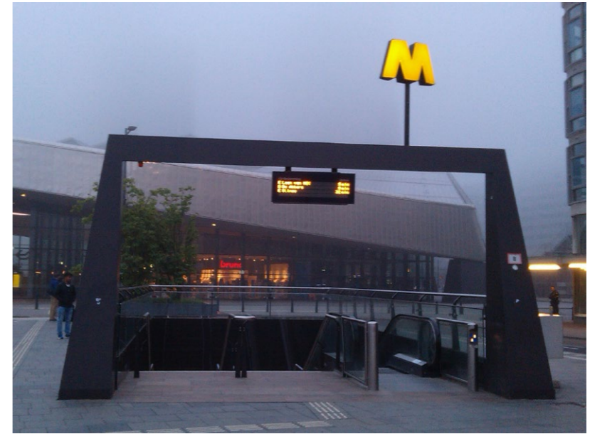
Figure 83. Multi-modal hub functions 24 hours, Rotterdam Centraal. How would city edge hubs be experienced? Photograph by author.
