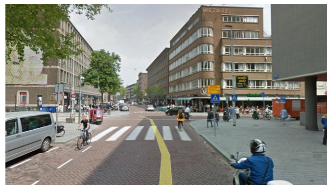
Figure 113. View on secondary street Meent. Google Street View.
