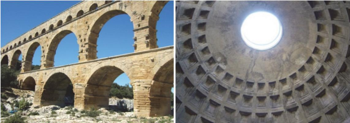
**Figure 1.1.** Pont du Gard and Pantheon Dome. Both of them have been surviving for two millennia proving engineering sustainability. The master builder design and built based on the knowledge that concrete is good in compression. Resisting solely compression, the dome needs no steel reinforcement which means no corrosion taken into account.
