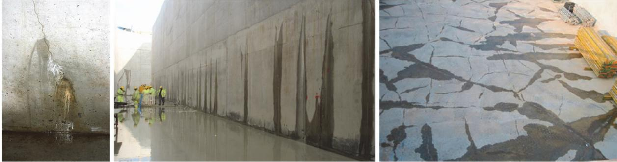
**Figure 1.2.** Cracks in concrete structures lead into unacceptable leakage and costly repair.
