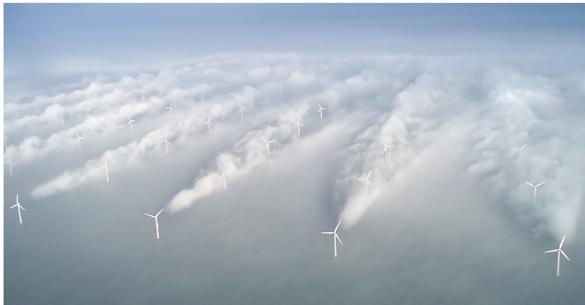
Figure 1-1: Photography of Horn Rev 1 offshore wind farm [2].
