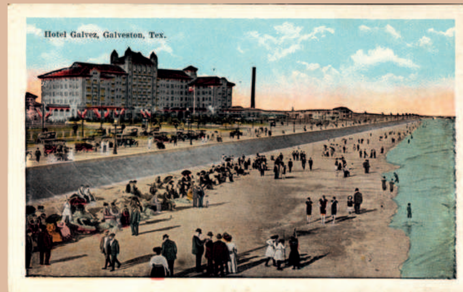
Figure 1. Multifunctional use of flood protection structures is not strange to Texas. The Galveston Seawall, here depicted on a postcard dating from 1911, was built with a road and hotels on top, as a response to the 1900 Great Hurricane (image courtesy University of Houston Digital Library).
