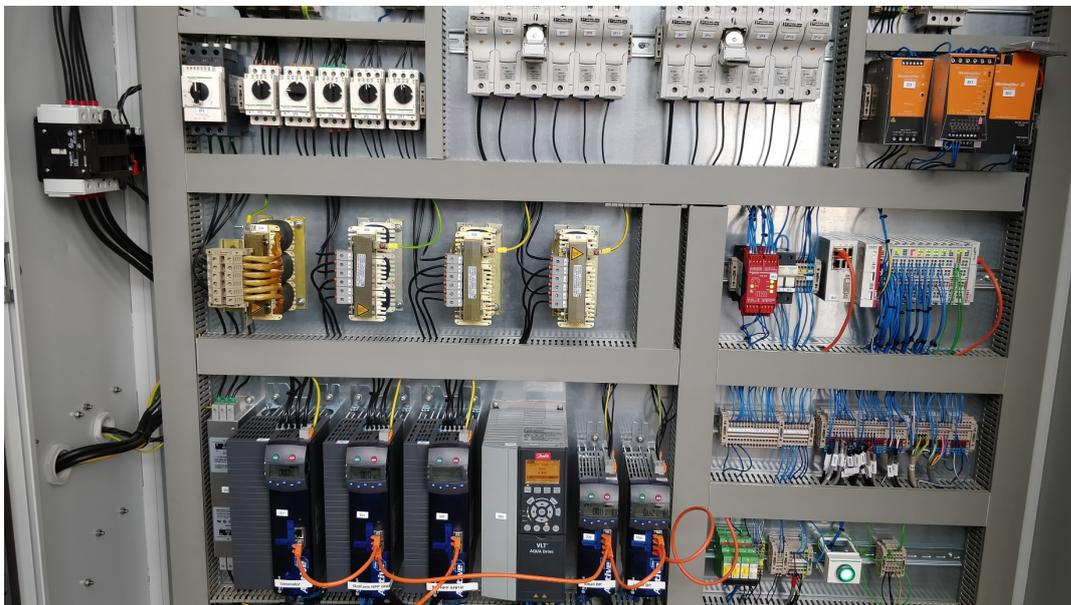
Figure 5.7: The electrical cabinet, containing the electrics and control hardware.
