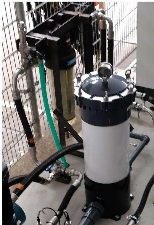
Figure 5.6: Cintropur  $10 \mu\text{m}$  filter(left) and EWP-USA  $3 \mu\text{m}$  filter (right).
