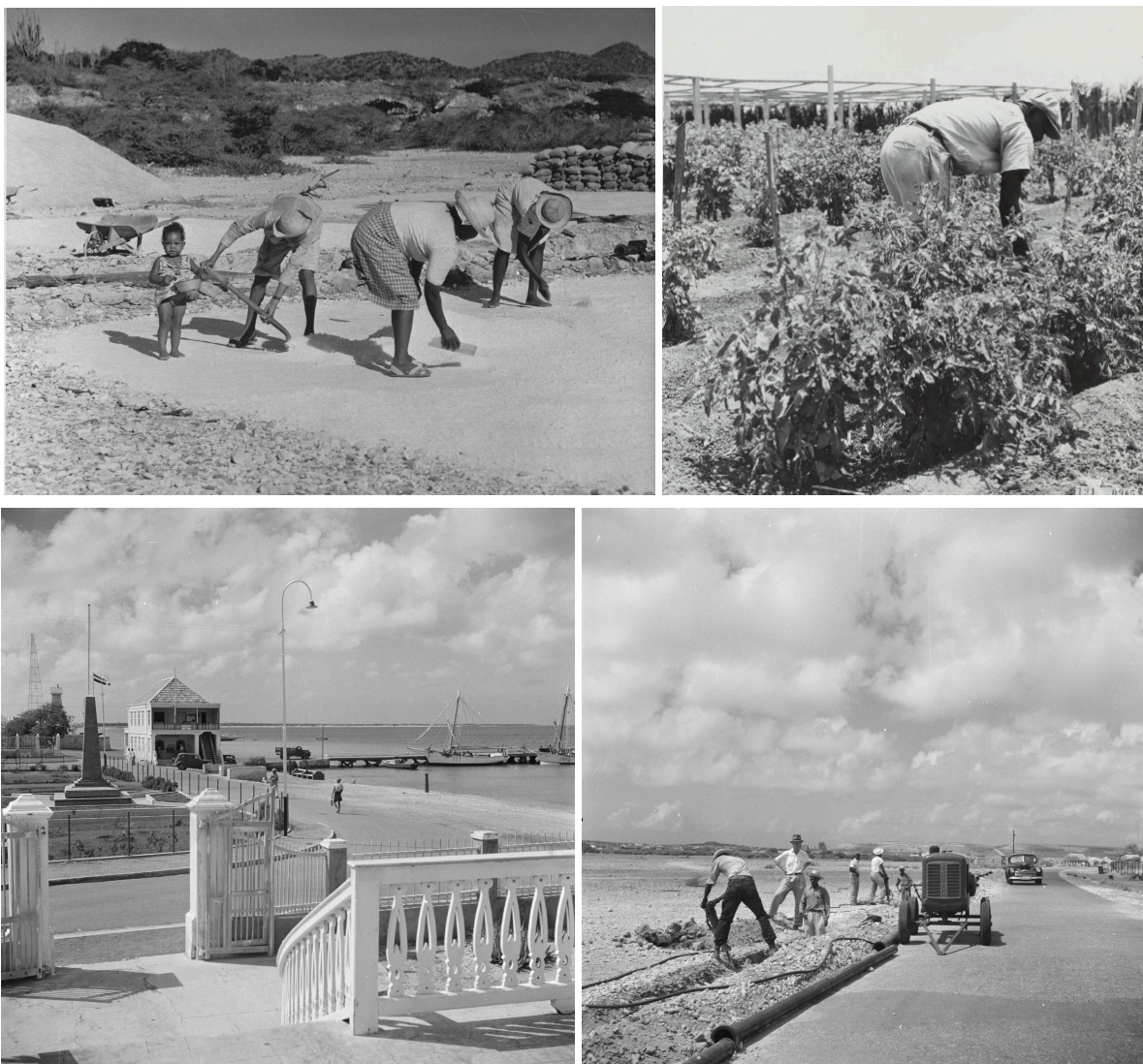
Figure 5.1., 5.2., 5.3. & 5.4. The top images show indigenous/freed slaves working on salt pans & agricultural land. Bottom images shows asphalt roads in and around Kralendijk (left: Wilhelminaplein, right: road towards salt pans). Source top left: Nederlands West-Indië. Bonaire. Zoutwinning, 1930s. Source top right: KITLV, 1940s. Source bottom: van de Poll, 1947.
