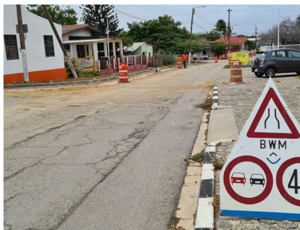
Figure 5.7. Road around Rincón. Source: Openbaar Lichaam Bonaire 2021b.
