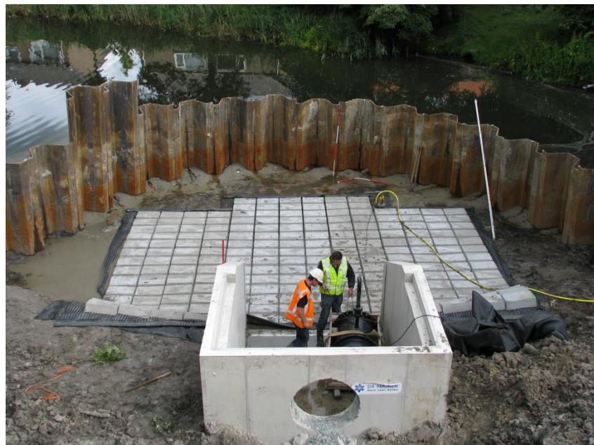
Figure 2.12 Installation of block mattresses (Holcim)
