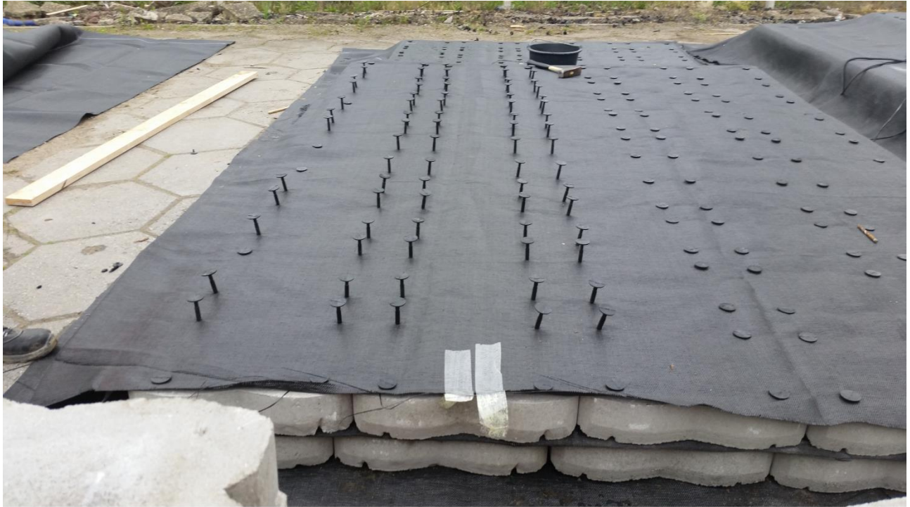
Figure 2.8 Placing plastic pins to connect the blocks with the geotextile
