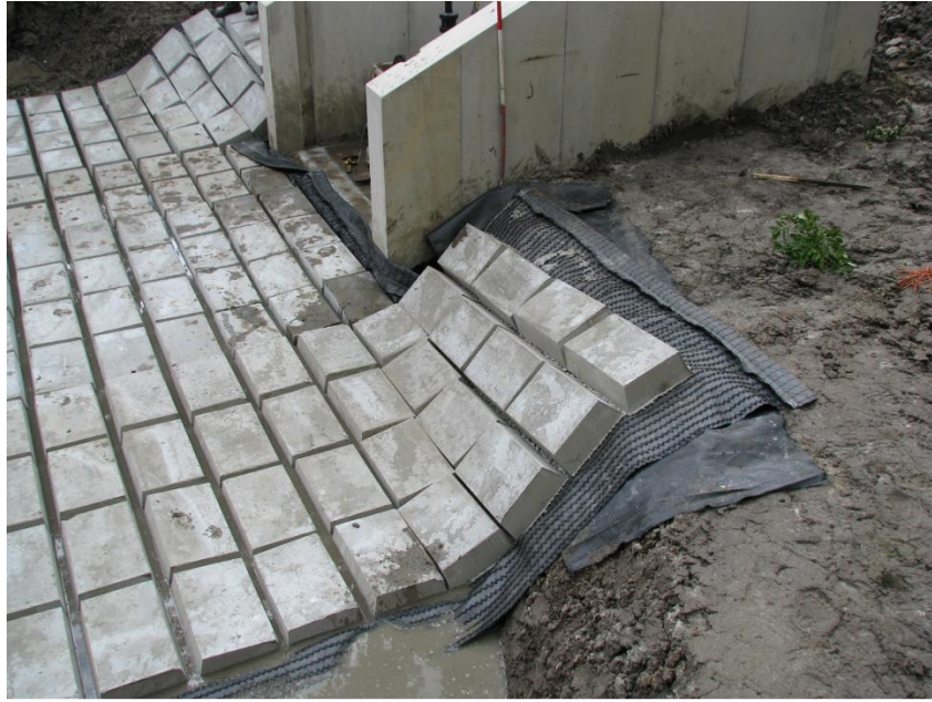
Figure 2.13 Direction of placed block mats (Holcim)
