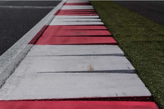
Figure 16.1.1: Ribbed kerbs (view is opposite from riding direction) (Flickr, n.d.).
