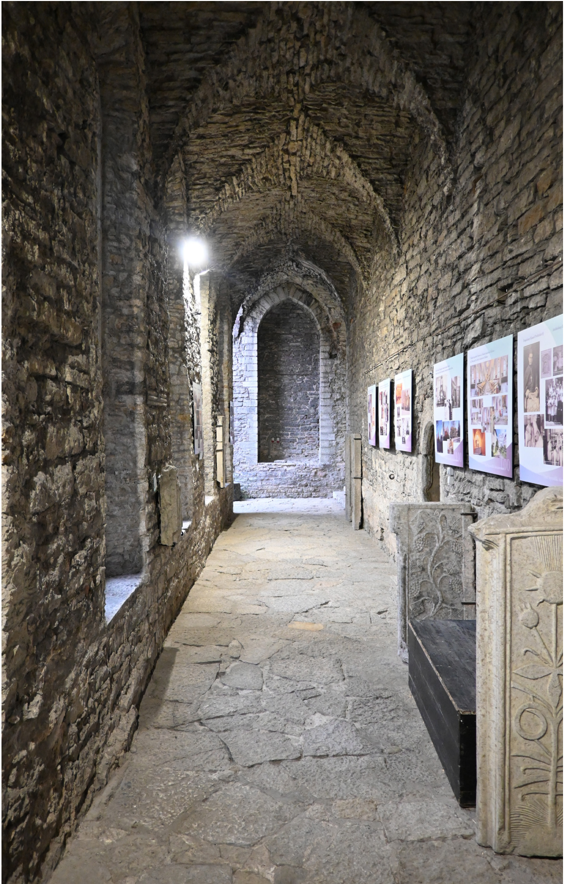
Image of the cloister hall as found
