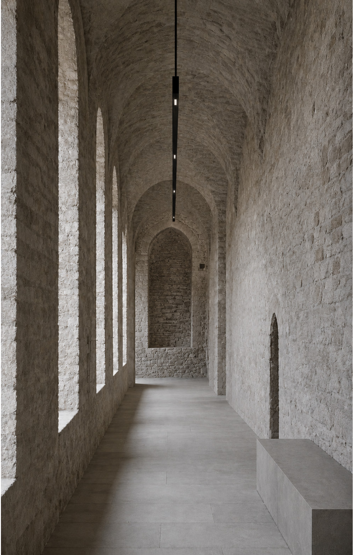
Render of the cloister hall after restoring
