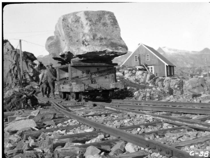
Figure 28. A some 20 tons block on a rail wagon. NCA
