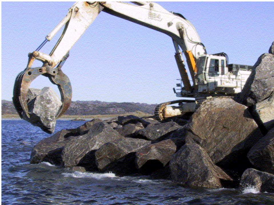
Figure 41. Placement of cover blocks on the Sirevåg berm breakwater. NCA.
