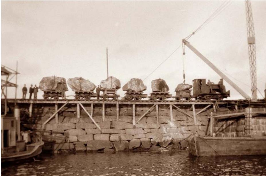
Figure 30. A train with breakwater blocks. NCA.
