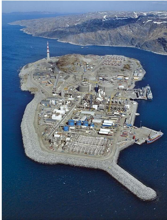
Figure 42. Melkøya LNG plant with the berm sea wall and berm breakwater. Photo: Eiliv Leren.
