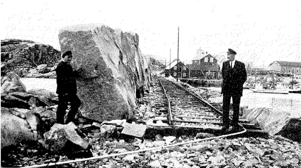
Figure 32. Crown stones placed on the Henningsvær breakwater.
