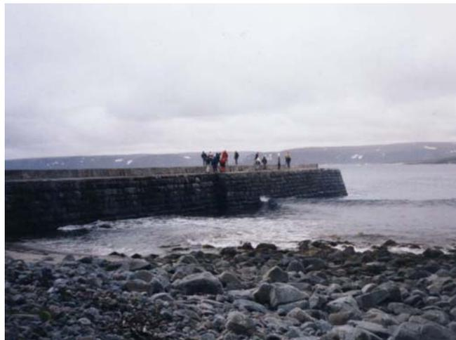
Figure 20. Blockwork breakwater at Hamningberg, Finnmark. Johnsen (2003).
