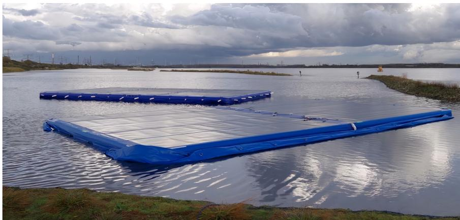
Figure 1.4: A photograph of the drop-stitch floaters of the Solar@Sea II project (courtesy of TNO).
