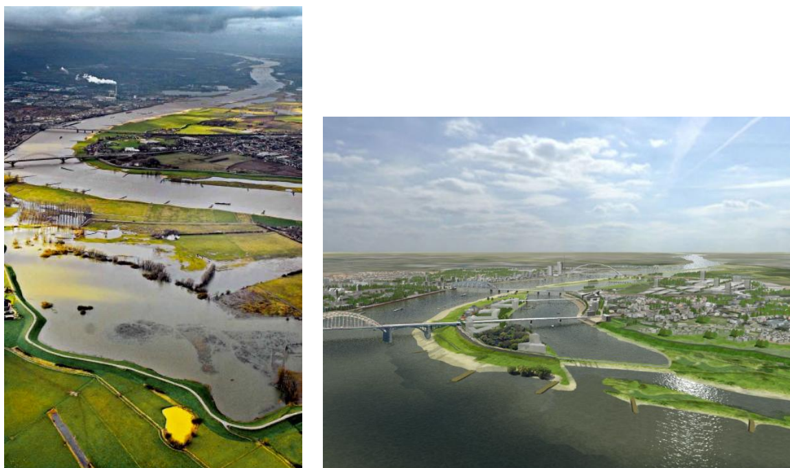
Figure 2.13 Example of one of the hydraulically most effective measures, which thanks to its eminent design team also greatly enhances the spatial quality, through – among other things – a second waterfront for Nijmegen city's north bank, larger recreational potential (boulevard, event terrain, beaches, rowing course), and better ecological connectedness of floodplain ecosystems. Present situation (left) and future situation (right).
