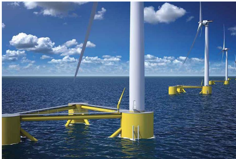
Figure 3.9: Offshore floating wind turbine including its foundation, on top of which the compressor station could be potentially placed
