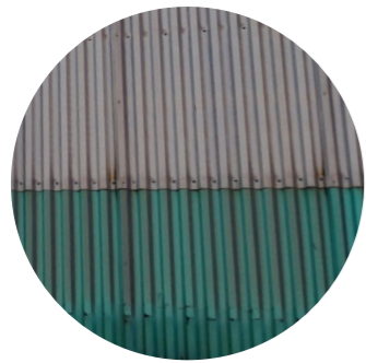
Coloured corrugated steel facade
