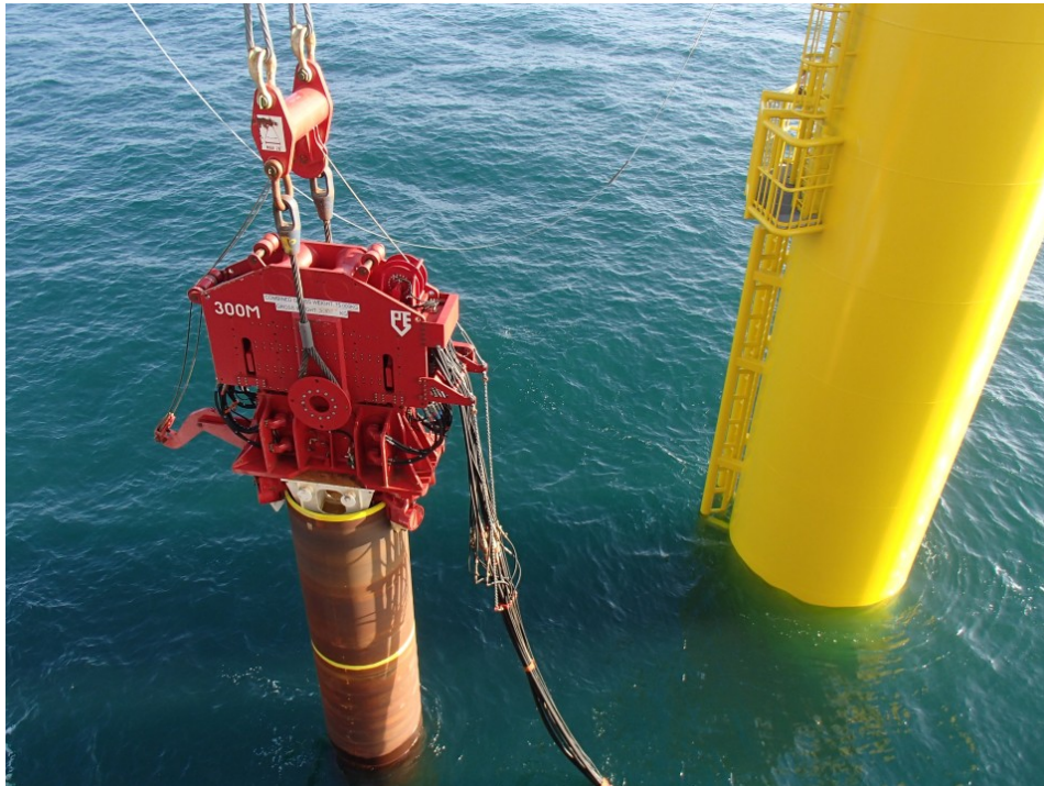
Figure 1.7: Vibratory hammer installation of pile in offshore environment (taken from [24])
