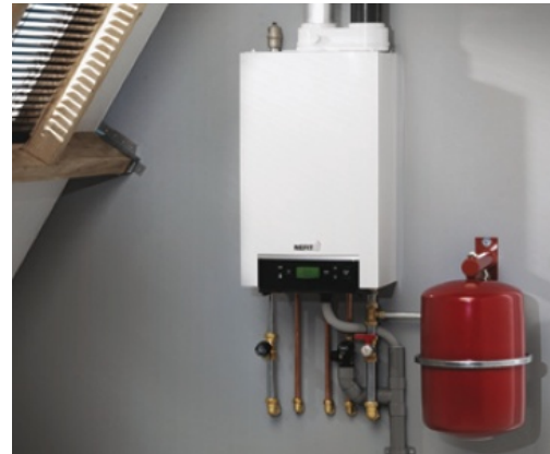
Figure 4-10: HR-Ketel positioned in attic Source http://www.van-trigtinstallaties.nl/site/cv-ketel-onderhoudscontract
