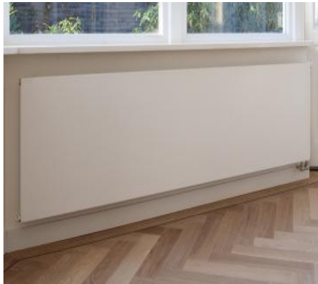
Figure 4-9: Standard radiator for heating distribution Source: http://www.adurad.nl
