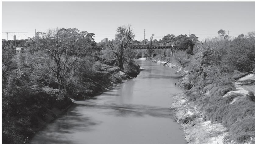
in 40.9 km (25.4 mi) of channel improvements (i.e., widening and deepening the main channel) and 22 km (13.7 mi) of concrete-lined channel DS of US-59 (HCFCD, 1998). At the time, the channel improvements were designed to provide enough capacity to
