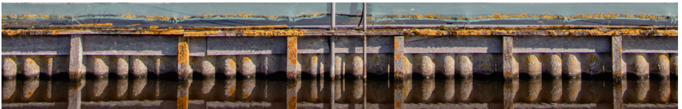
↑ Schoeiing with corrugated sheets
