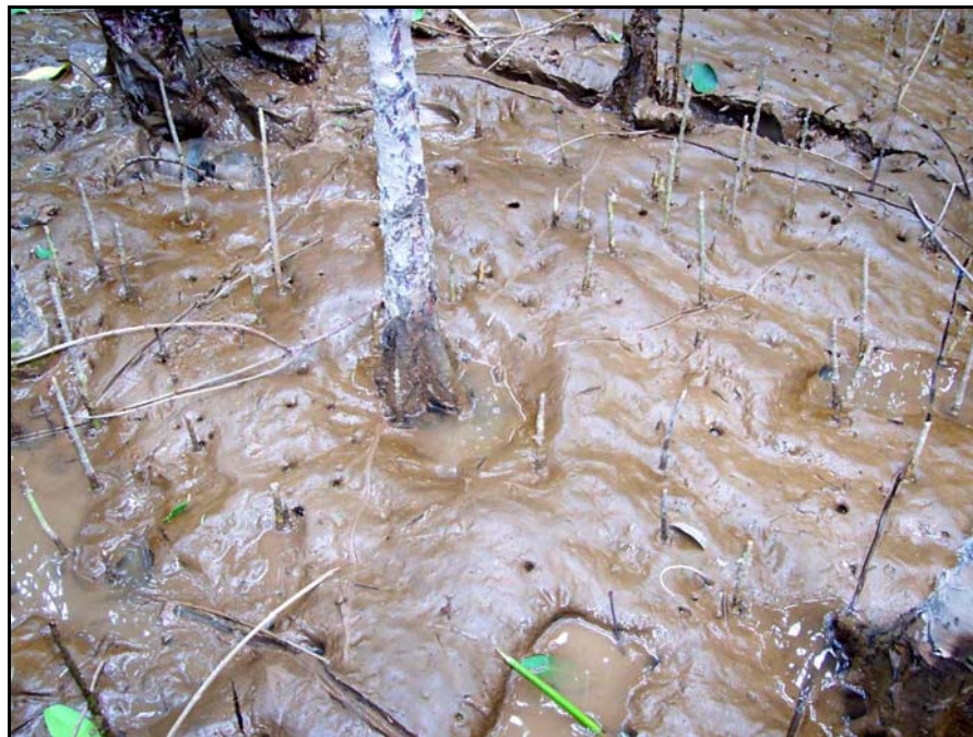
Figure 9.3 Scour hole at tree base and disturbance by humans
