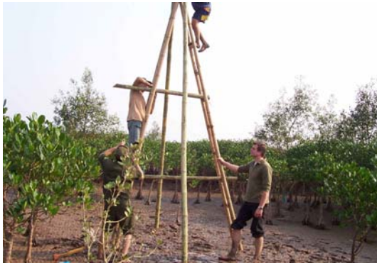
Construction of tower
