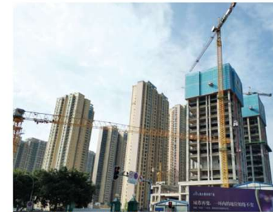
Image 18. the construction of high-rise community in CAOJIAXIANG, 2017
