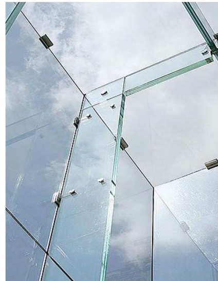
Bolted connection
