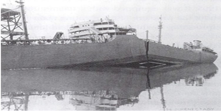
Figure 1.1. T-2 tanker fractured in 1943 [3].
