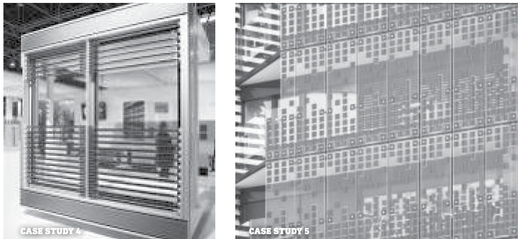
FIG. 2 The positioning of opaque energy-harvesting elements is usually designed not to obstruct the view: From left to right: A. Façade prototype: "Solarthermie in the Fassade". The Institute for Building Construction and Design III (2008, exhibited at Glasstec 2008). B. Lyon housing Hikari (arch. Kengo Kuma, 2015). Photographs by the author.
