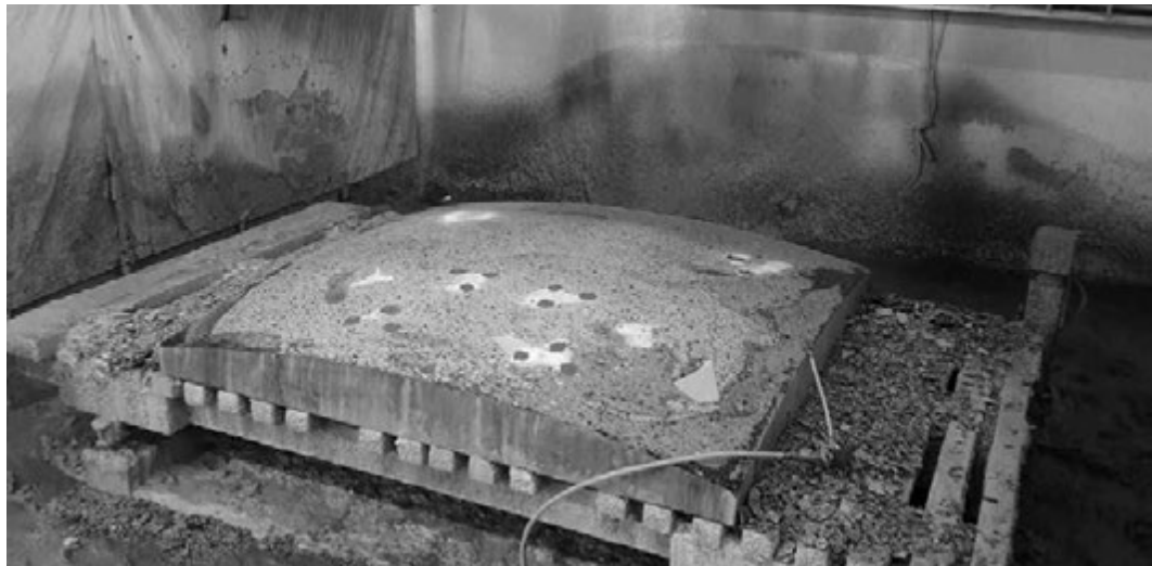
FIG. 14 Concrete Formwork Fabrication with a 5axis CNC Milling machine
