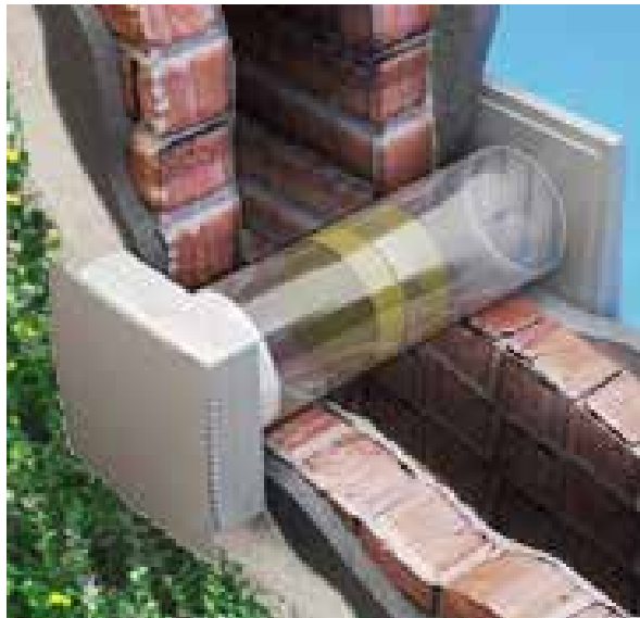
FIG. 6 Example of a fresh air inlet device
