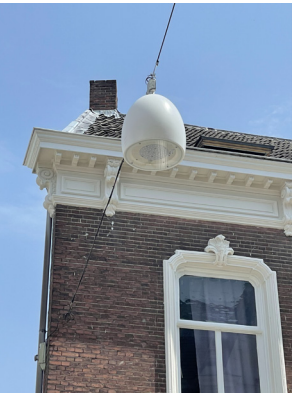
mmWave radio aesthetically integrated into a luminaire fixture
