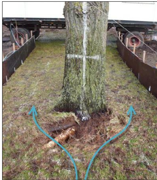
Figure 3-2: Erosion pit in front of a tree during the field experiment at the Vechtdijk (Bakker et al., 2010)
