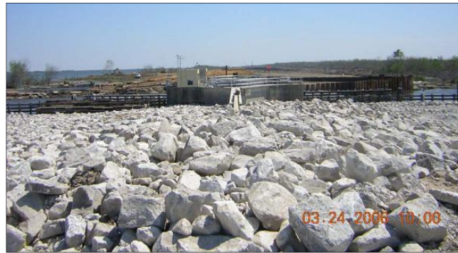
Figure A-8: The transition has been reinforced with rip-rap. (picture: Rune Storesund)
