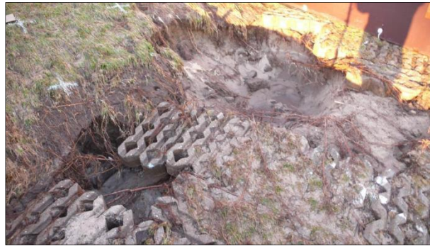
Figure B-2: End result at the first test slope
