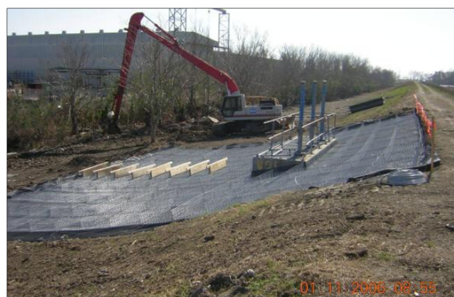
Figure A-7: Dike protection work of soil-structure interactions (picture: Rune Storesund)
