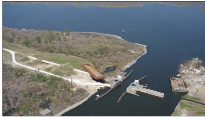
Figure A-3: The dike transition suffered from severe erosion (picture: Les Harder)
