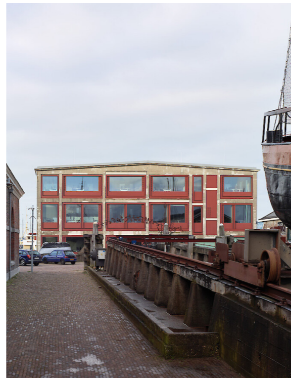
Figure C.3. City Hall Den Helder by Office Winhov. Source: https://www.winhov.nl/
