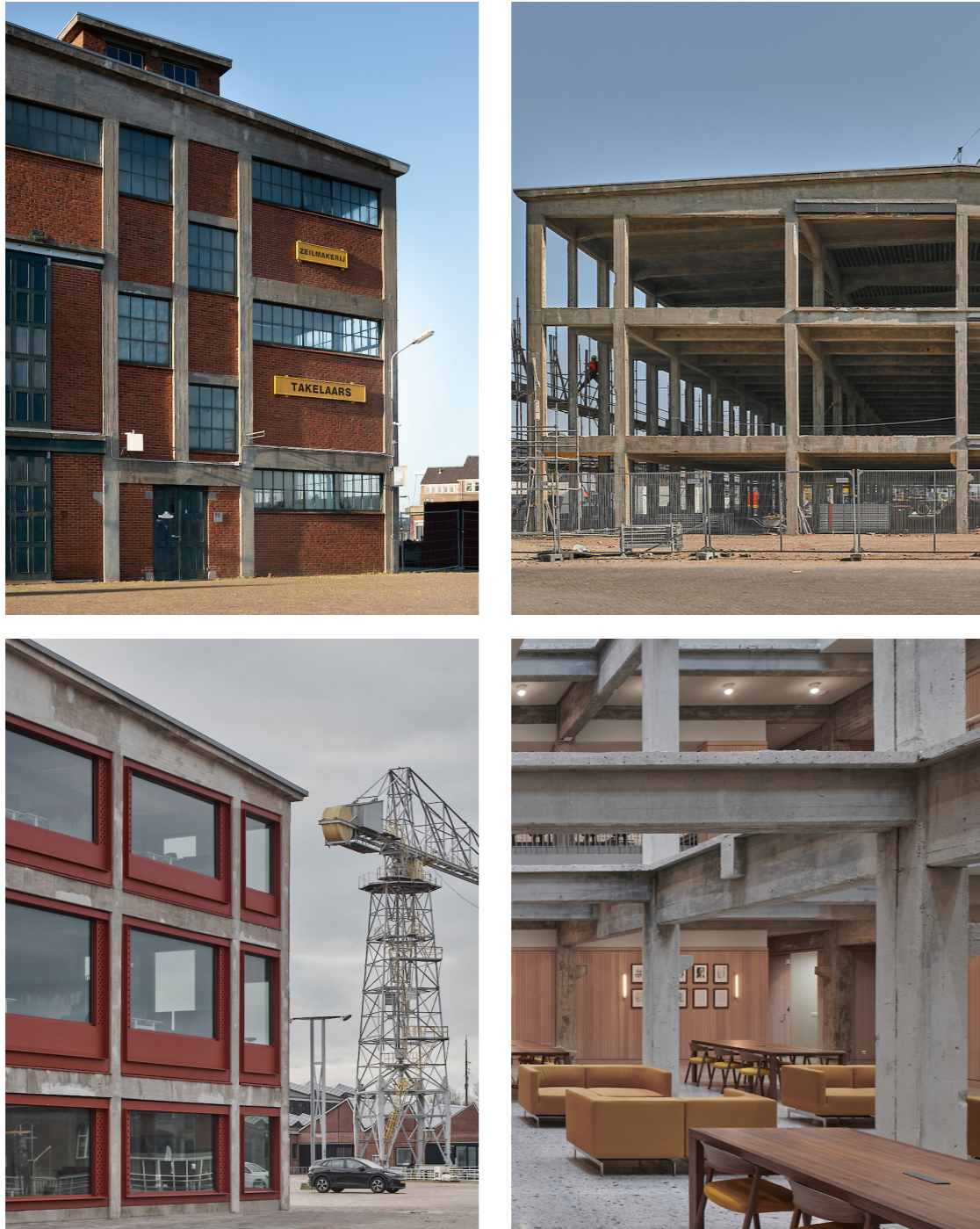
Figure 21. Selection of images of City Hall Den Helder, from left to right; original building, uncovering identity, reconstruction with catalogue and pallet, and interior as palimpsest. Source: Office Winhov (2024)
