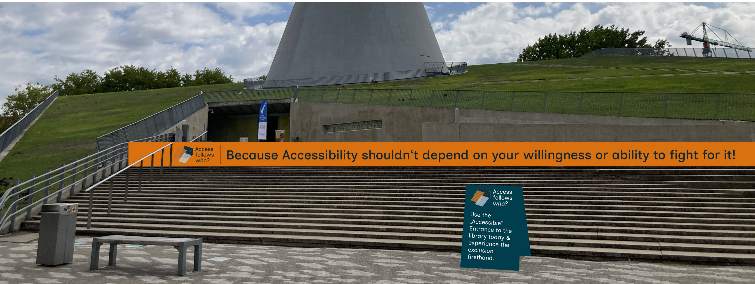
Fig. 52: Blocked Entrance at the Library
