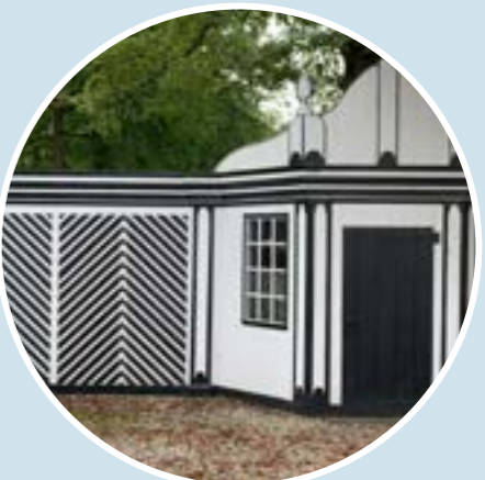
HUIS 't VELDE WARNSVELD Wooden planks Reused for facade cladding
