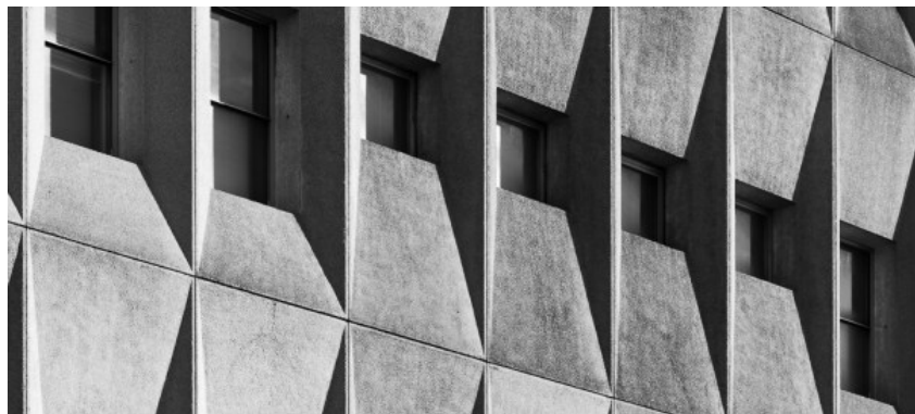
Figure III.V. Smooth concrete surfaces on precast concrete elements. Source: Miners, N.
