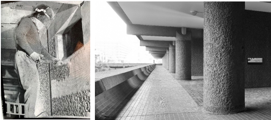
Figure III.X and Figure III.XI. Bush-hammering employed in the Barbican Estate, London. Sources: Barbican Living.; The Modern House
