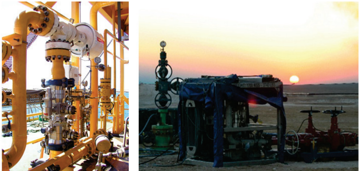
Figure A.5: Example of a permanent installed Vx meter (PhaseWatcher) and mobile Vx meter (PhaseTester).
