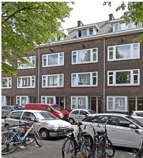
A cluttered sidewalk in Tarwewijk where parked bicycles, and nearby cars obstruct pedestrian access, highlighting a conflict of functions that compromises mobility and accessibility (own image)
