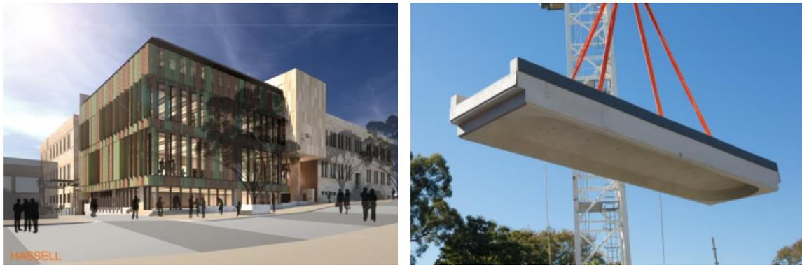
Fig. 2.11: Render of the Global Change Institute (left) and at the right a geopolymer concrete beam, with a length of 10.8 meters, being craned into position (Aldred & Day, 2012, p. 14).
