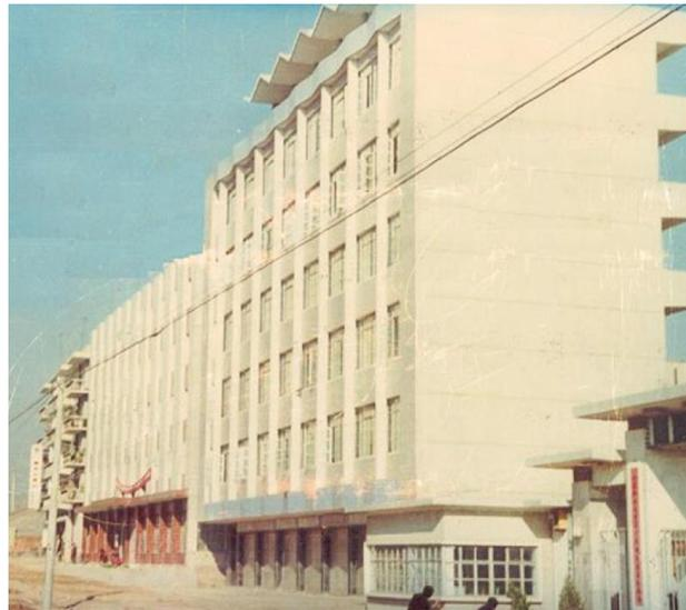
Fig. 2.10: 6-storey building in Kraków, built with alkali-activated slag concrete in 1974 (J. L. Provis, Brice, et al., 2014, p. 314)
