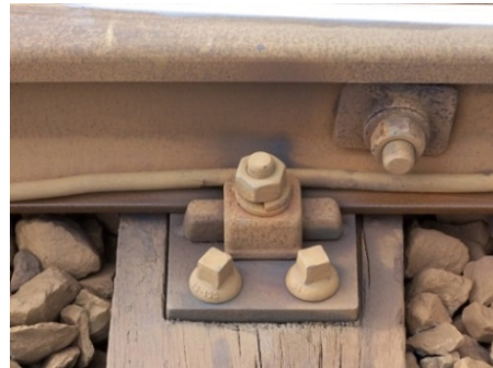
(f) Indentation of baseplate into sleeper
