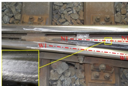
Figure 5.11: Repaired crossing profile with a magnified image of grinding marks
