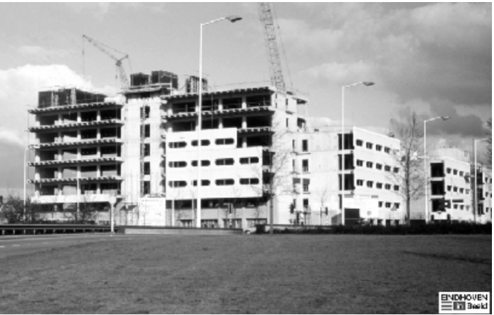
Figure 5: A picture of the WTC office building in construction (Eindhoven in Beeld, 2010)
