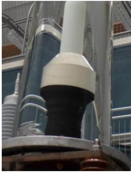
Figure 17: Stress cone of a cable termination
