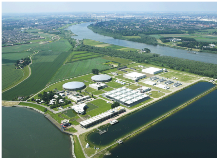
Figure 1.6. Water treatment plant in the Netherlands.
