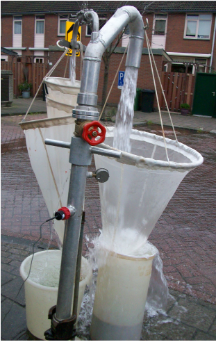
Figure S4.1. Mains flushing. A fire hydrant is opened and using a high flow rate, water together with sloughed biofilm, loose deposits, and suspended solids are collected.
