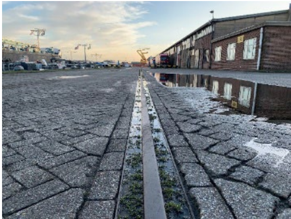
Figure 21: Tracks of the rocker cranes (Source: photograph taken by the author on March 14, 2023)
