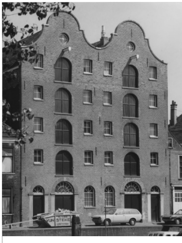
Figure 1: Den Dubbelde Palmboom after the renovation of 1975 (Source: Stadsarchief Rotterdam)
