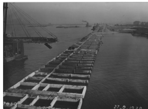
Figure 4: Caissons are used to construct Merwehaven (Source: Stadsarchief Rotterdam)
