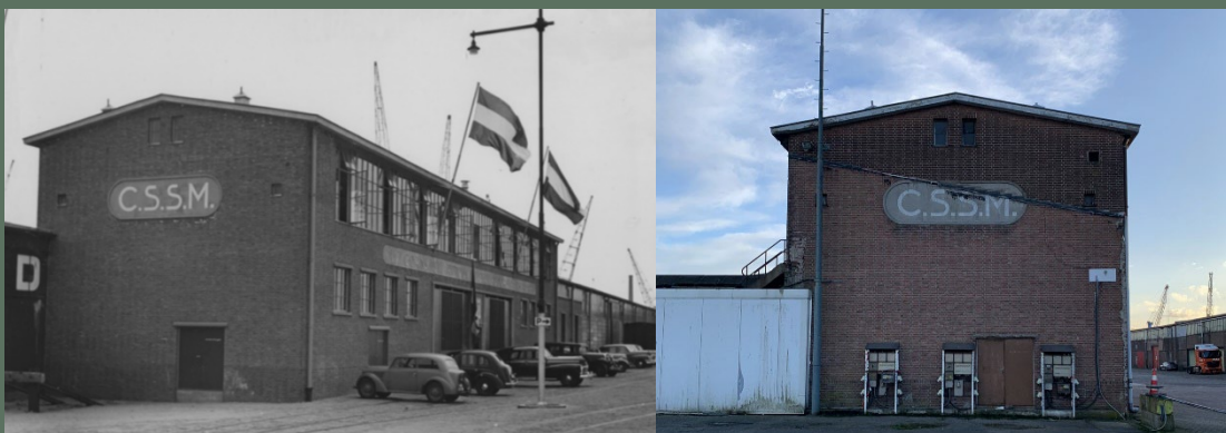
Figure 29: office building C.S.S.M. (Source: Stadsarchief Rotterdam, courtesy of Mr. D. van de Ven)
