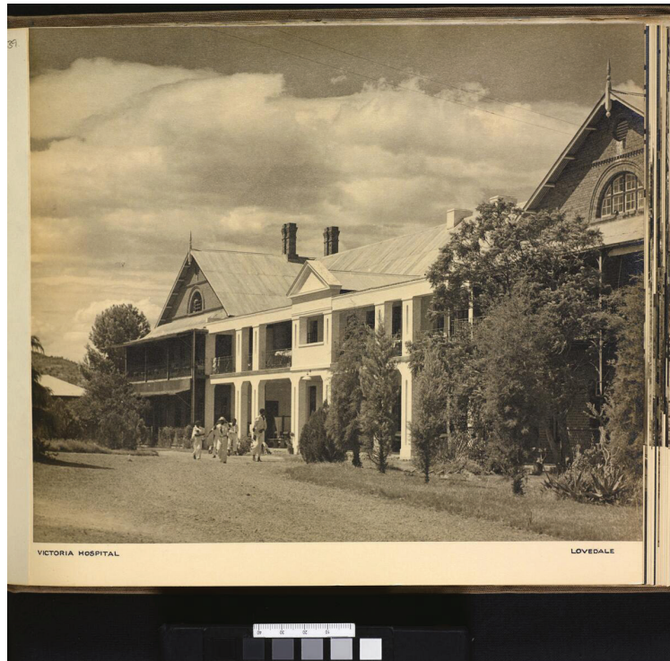
Figure 3.2.3 Victoria Hospital National Library of Scotland (1938)
