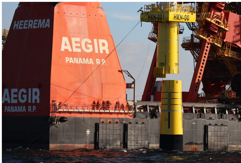
Figure 1.3: Installation of a slip joint monopile (DOT, 2025).
