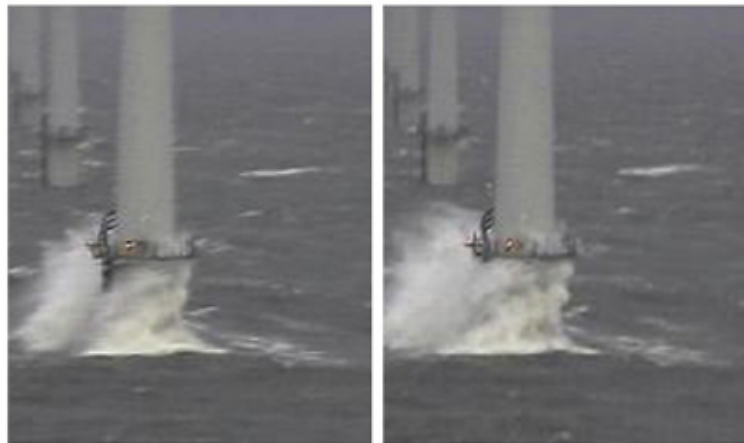
Figure 1.1: Wave run-up at Horns Reef 1 for H_s \approx 2.5 m, while the platform level is 9.0 m above MWL. H_{s,design} = 5.3 m (Lykke Andersen et al., 2011).
