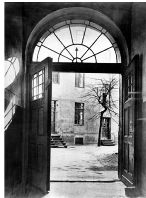
Figure 147: View at the Siemens & Halske workshop at Schöneberger Strasse in Berlin (1847).
