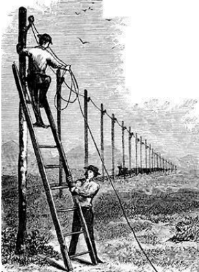
Figure 179: Telegraph lines installed on poles along the rail tracks.
