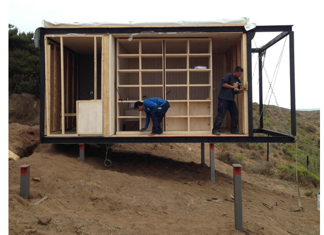
Figure 13. Remote House during installation.
