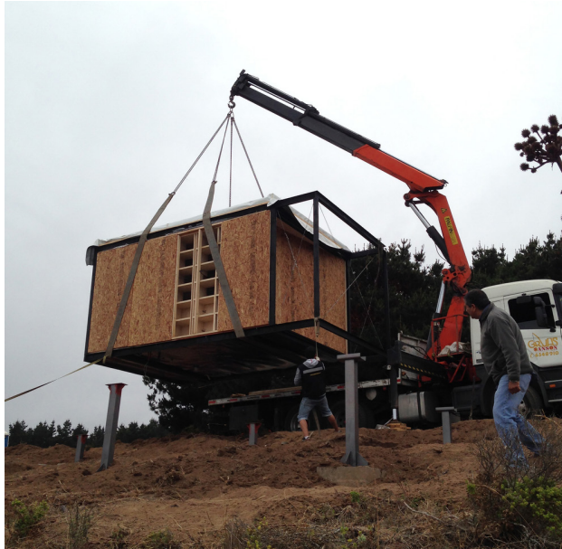
Figure 12. Remote House during transport and assembly.
