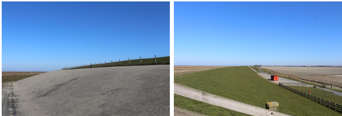
Figure 4-4: Holwerd sea dike slopes. Seaward side ( left ) and Landside ( right )
