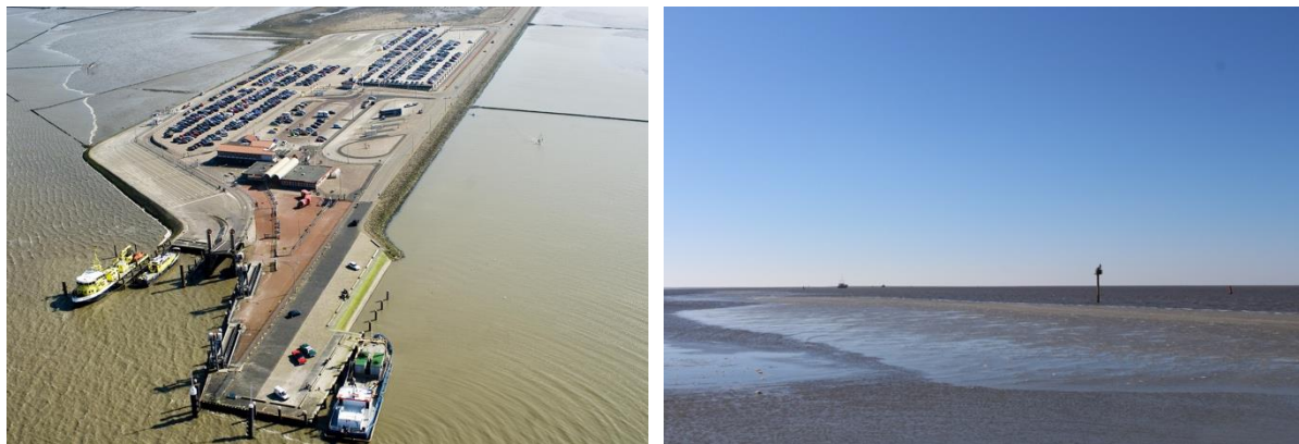
Figure 4-6: Ferry terminal ( left ) and navigation channel ( right )
