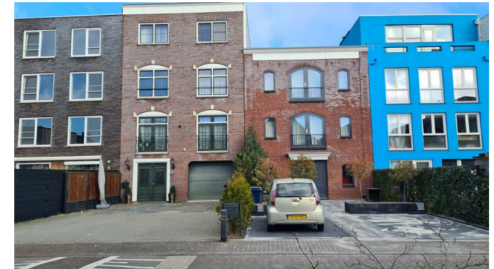
Figure 4.33: Distinctive architectural expression, Aresstraat
