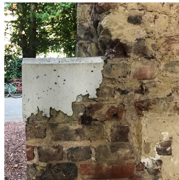
Figure 5.1. Patching the corner with concrete.
