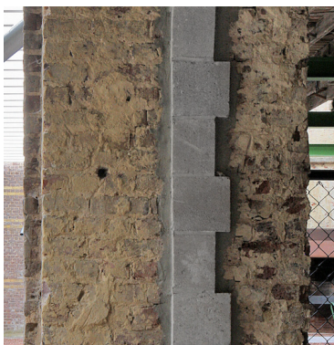
Figure 5.3. New concrete blocks restructure the brick wall.
