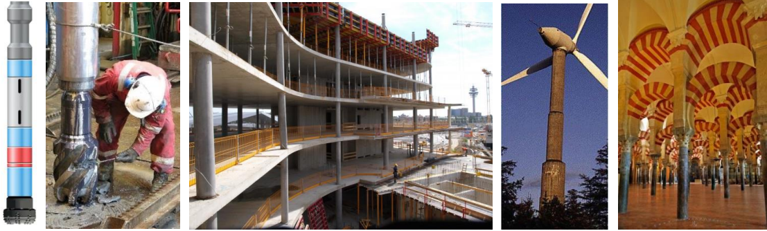
Figure 1: Examples of physical structures that can suffer from instability. (a) drill-strings under high compressive loads and consisting of many elements of different cross-sections. (b) structural columns that have different material properties at the column-slab-column interface. (c) stepped wind turbine subjected to high lateral loads. (d) structural columns with step-changes in their cross-section.
