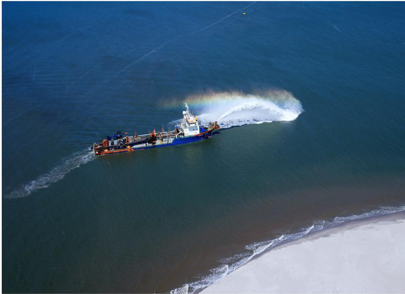
Figure 1.3: Coastal reinforcement near The Hague by application of rainbowing. In this process the sand-water mixture is collected from the sea-floor and transported to the coastal region. The rainbowing process allows deposition of the slurry in shallow water areas. Figure taken from “Beeldbank Rijkswaterstaat”.
