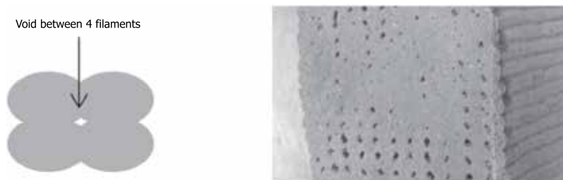
Figure 46 - Voids between printed concrete (concrete printing) (1)
