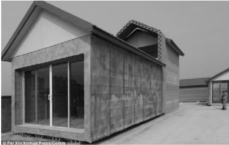
Figure 35 - Printed concrete house (2)
