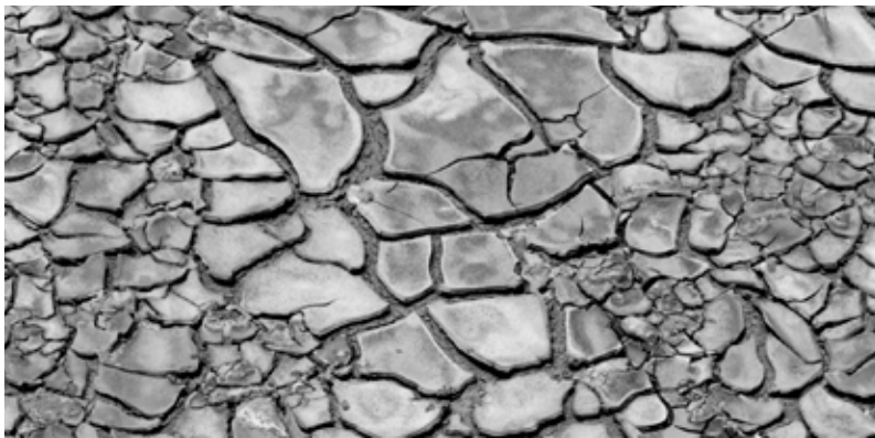
Figure 13 - Cracking of clay
