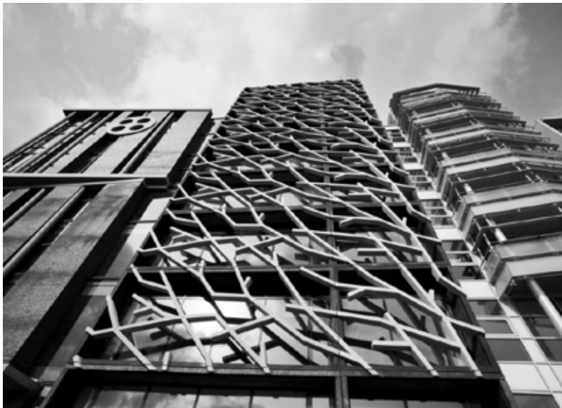
Figure 2 - Zilverparkkade concrete façade by René van Zuuk Architecten (1)
