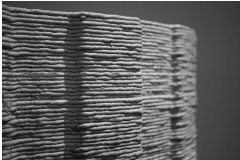
Figure 51 - Surface 3D-Concrete printing (1)
