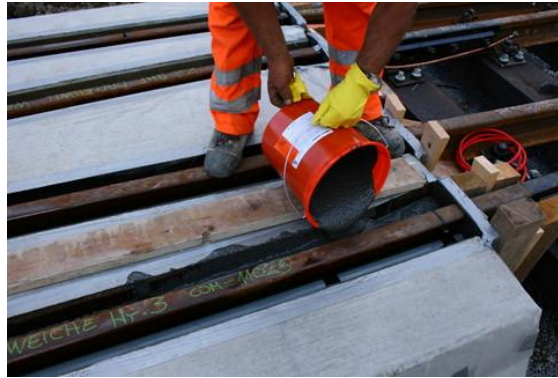
Figure 11: Pouring of Corkelast in-situ
