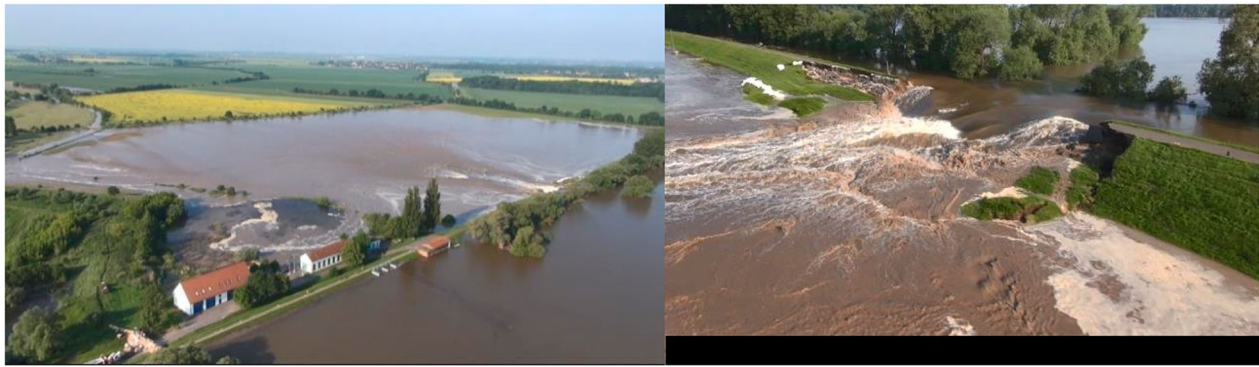
Figure 5. Left: overview photo of the inland while the flooding evolves, Right: overview photo of the breach at 10-jun-2013 (Grubert 2013; Weichel 2013).
