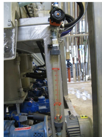
Figure M.12. Large water flow regulator.
