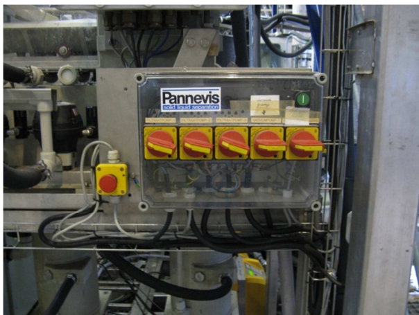
Figure M.11. The 'Pannevis switch box'. The green button is the reset. The red switches are from left to right; Filtrate Pumps 1 till 3, Vacuum Pump, Belt Filter Mains.
