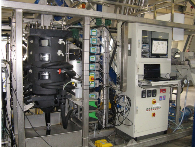
Figure 5.4. An overview of the 200 liter pilot plant. The insulated crystallizer is shown at the left.
