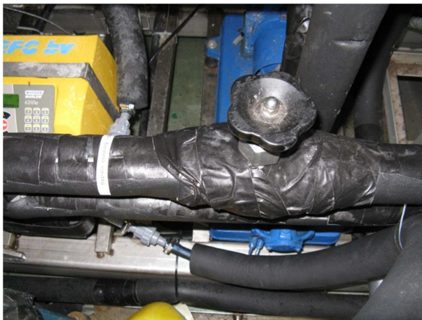
Figure M.5. Cooling liquid by-pass valve.
